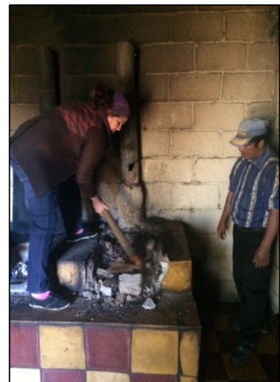
Dismantling Outdated Cookstove
